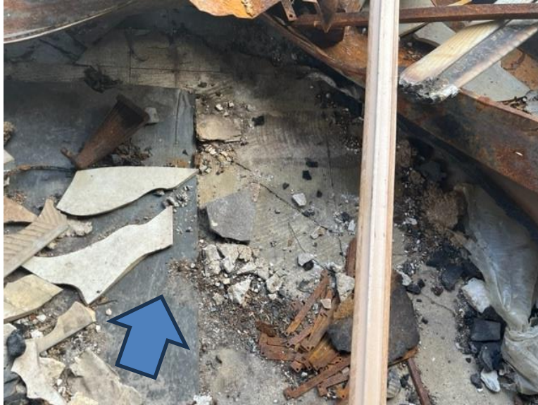
Photograph 1: Showing an example of the asbestos blue vinyl sheet flooring located at the Site.
