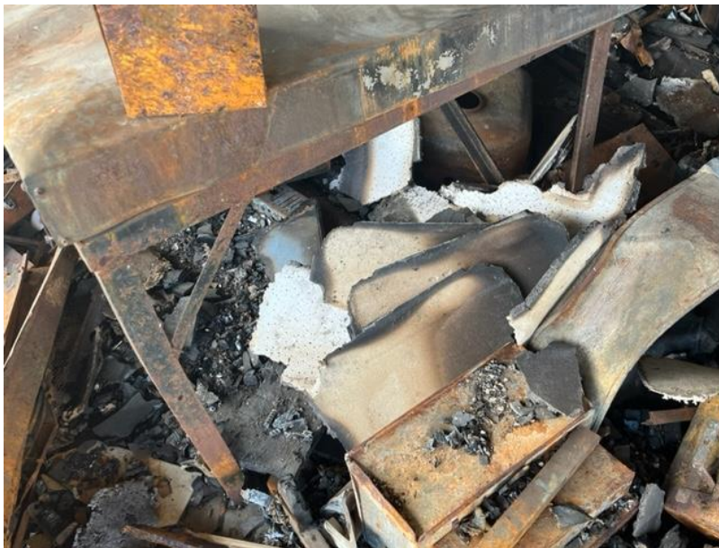
Photograph 4: Showing an example of the non-asbestos ceiling tiles located at the Site.
