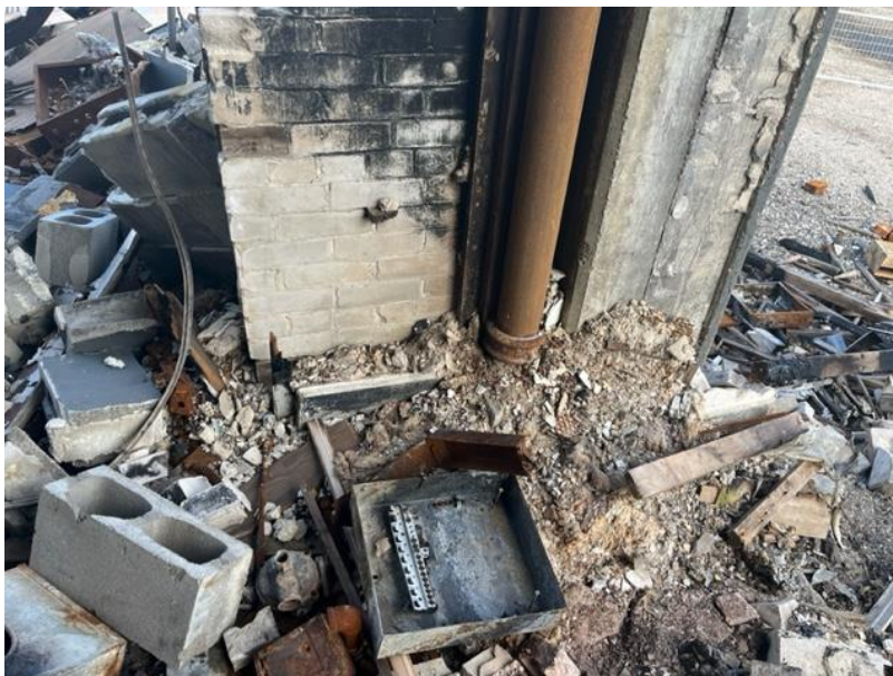
Photograph 6: Showing an example of the non-asbestos brick mortar located at the Site.
